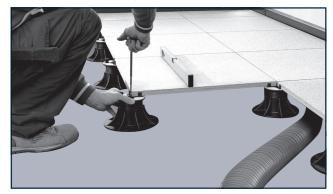
The adjustable supports offer multiple solutions to compensate for small imperfections and large slopes on any laying surface and to create perfectly stable floors with the correct slope.
