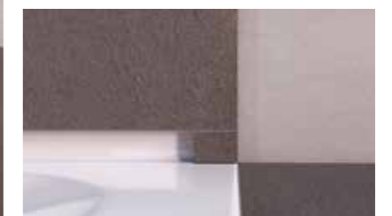
A small piece of tile is placed behind the shower screen in order to close the hollow space
