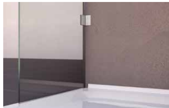
with shortened upstand and trimmed tile
