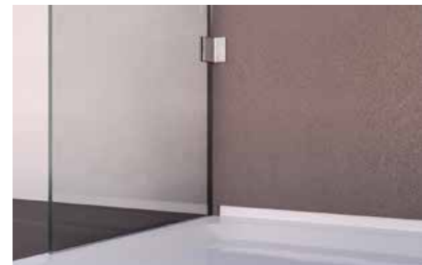
The hinge goes in front of the trimmed tile (no additional joints)
