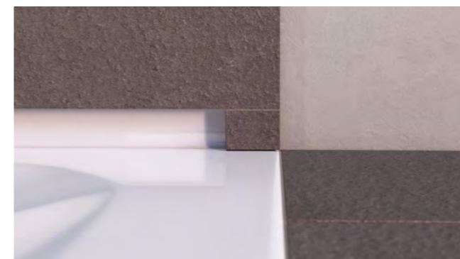
A small piece of tile is placed behind the shower screen in order to close the hollow space
